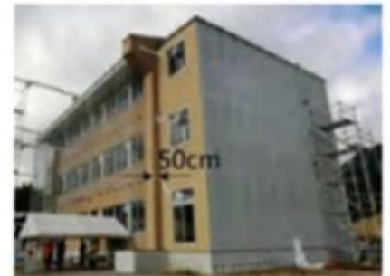
Fire wall (Final test)
